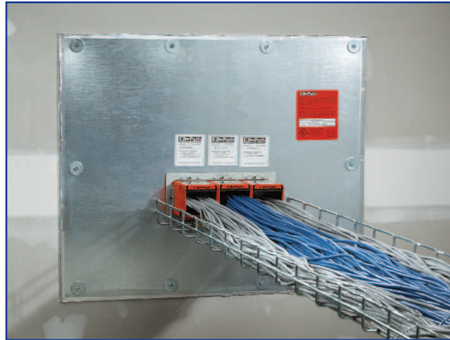
Large opening reduction with composite sheet and EZ-Path® Fire Rated Pathways.
